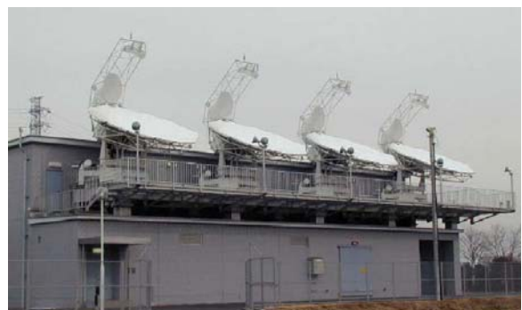
Uplink Center (secondary earth station: Shobu)
