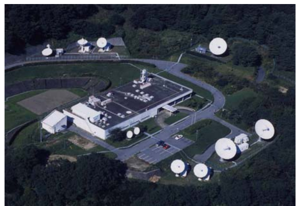
Kimitsu Satellite Control Station (unmanned backup station)
