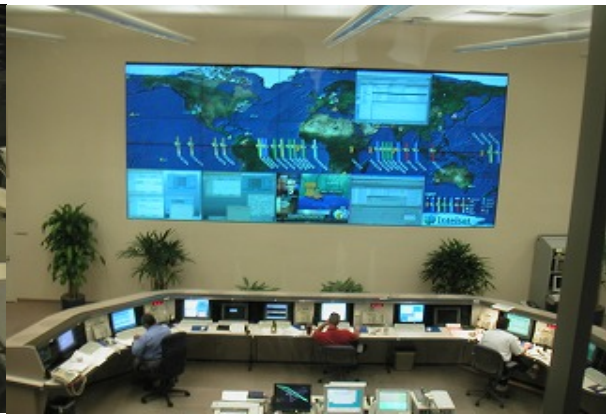
Communications Control Room
