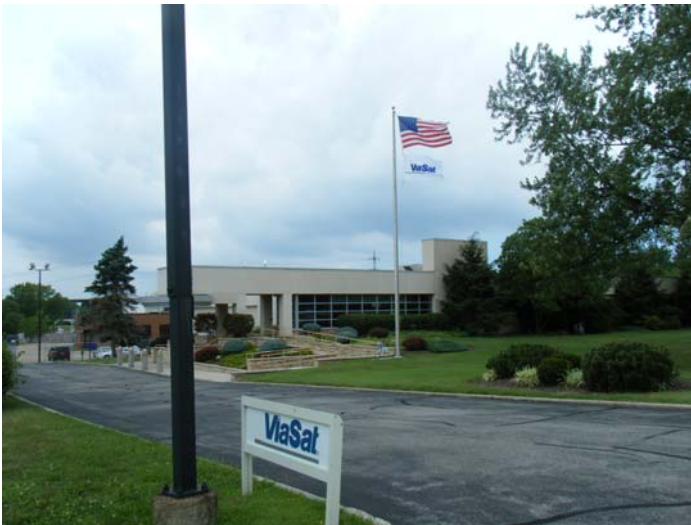
▲ ViaSat ECC Facility in Cleveland
