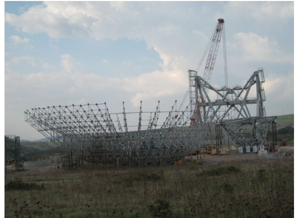
Saldinia radio telescope under construction.
