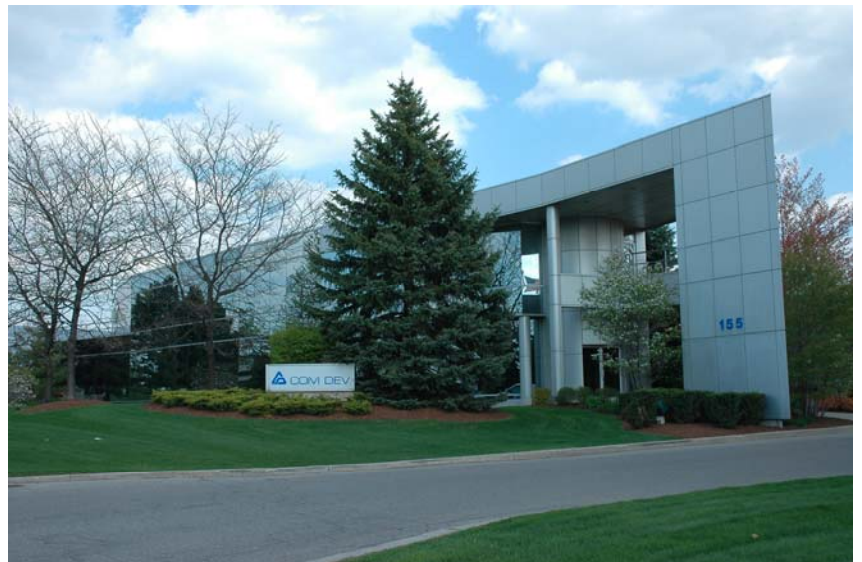
Fig. 2: Com Dev Facility at Cambridge
